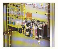
performance of the control unit. As a result of this and other design factors, a standard DC system will work over the temperature range of -20°C to +35°C without de-rating and to +55°C with de-rating. Any variation in output voltage and current are detected, processed and fed to the thyristor firing circuits which control the thyristor firing angle.
